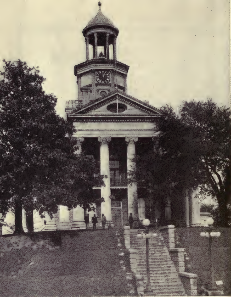
WARREN COUNTY COURTHOUSE, VICKSBURG
